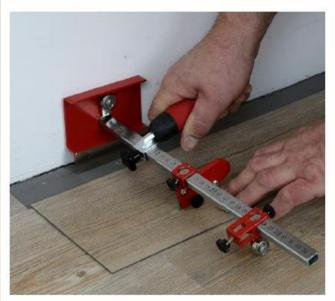
• Then align the floor tile to be trimmed with the last row of tiles laid and slide the precision edge trimmer while holding the stop parallel to the wall (the stainless steel edge of the stop must go into the adhesive bed). Lift the handle (3) slightly to score the surface of the covering (illustration 3). Then fold the covering down at the score mark and break.
